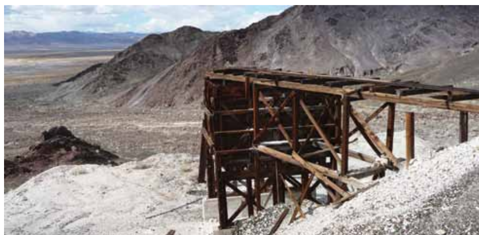
Decaying mine structures are hazardous.
