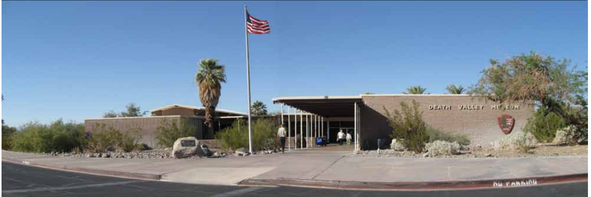
The rehabilitation of the Furnace Creek Visitor Center will make it more energy efficient.
